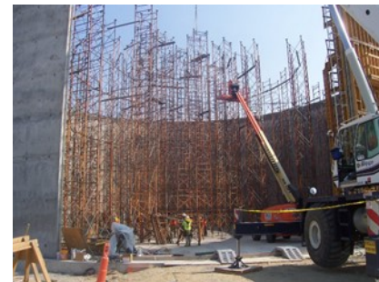
-Billings Water Tank Project, 2018
