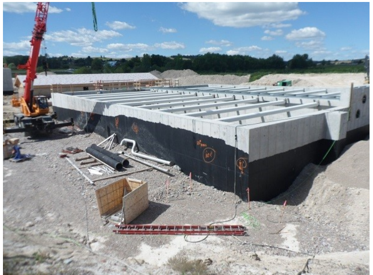
-Polson Wastewater Project, June 2018
